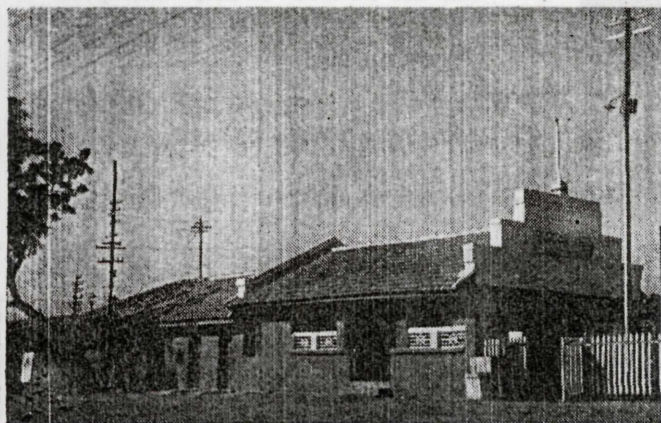
Old Station Building, Rourkela.
